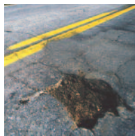
POTHOLE & BLOWOUTS
